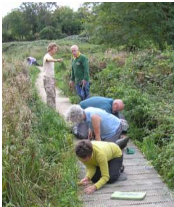
Fastening weldmesh to the surface of the boardwalk.
